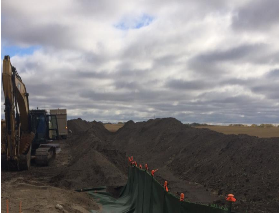
Topsoil stripping at 744 + 768
